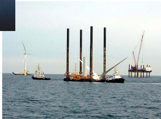
The 60-megawatt North Hoyle project off the coast of Wales is typical of today's offshore wind farms. Installed in May 2003, it consists of thirty Vestas 2-MW turbines, each having a rotor diameter of 80 meters. This project occupies an area of six square kilometers.
